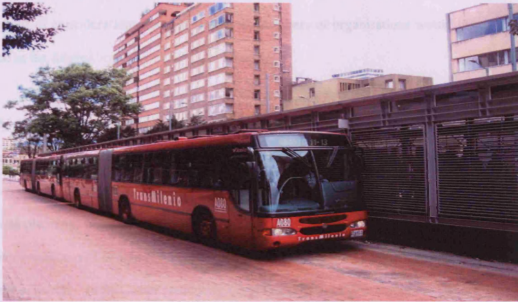
Picture 5. 'Trunk' buses in one of the platforms of the corridors.
